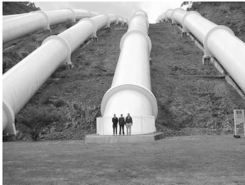
The six pipes ► of the power station Tumut 3 are each 487 meters long, 5.6 meters in diameter, and collectively contain 10,260 tons of steel.
