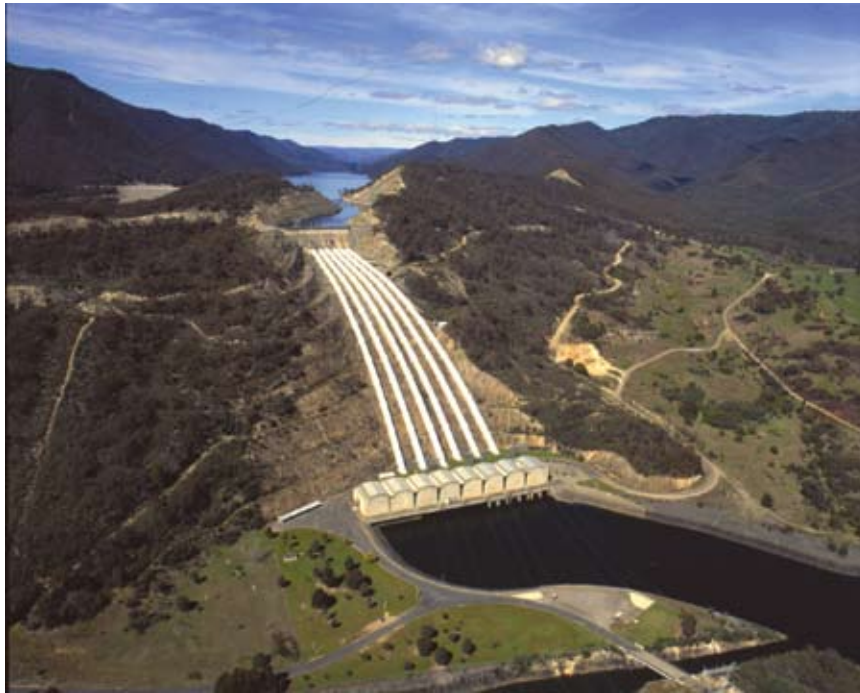
▲ Six generators at Tumut 3 power station. Two of them can provide enough electricity to power a city the size of Australia's capital, Canberra.
