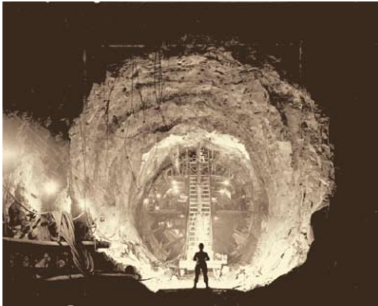
Construction ► at the Snowy Mountain Scheme's underground power station Tutmut 1, in 1958.
