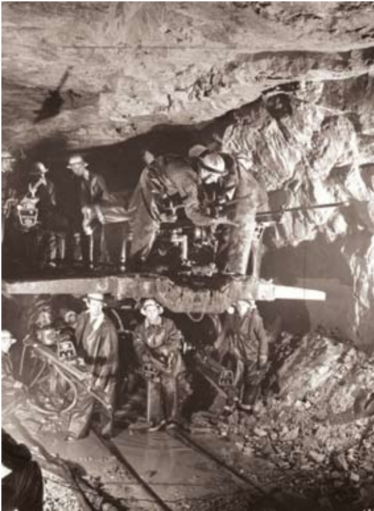
▲ Endersbee was a world authority on rock behavior and tunnelling. Here drilling at the Tooma-Tutmut tunnel, part of the Snowy Mountain Scheme, in 1959.
