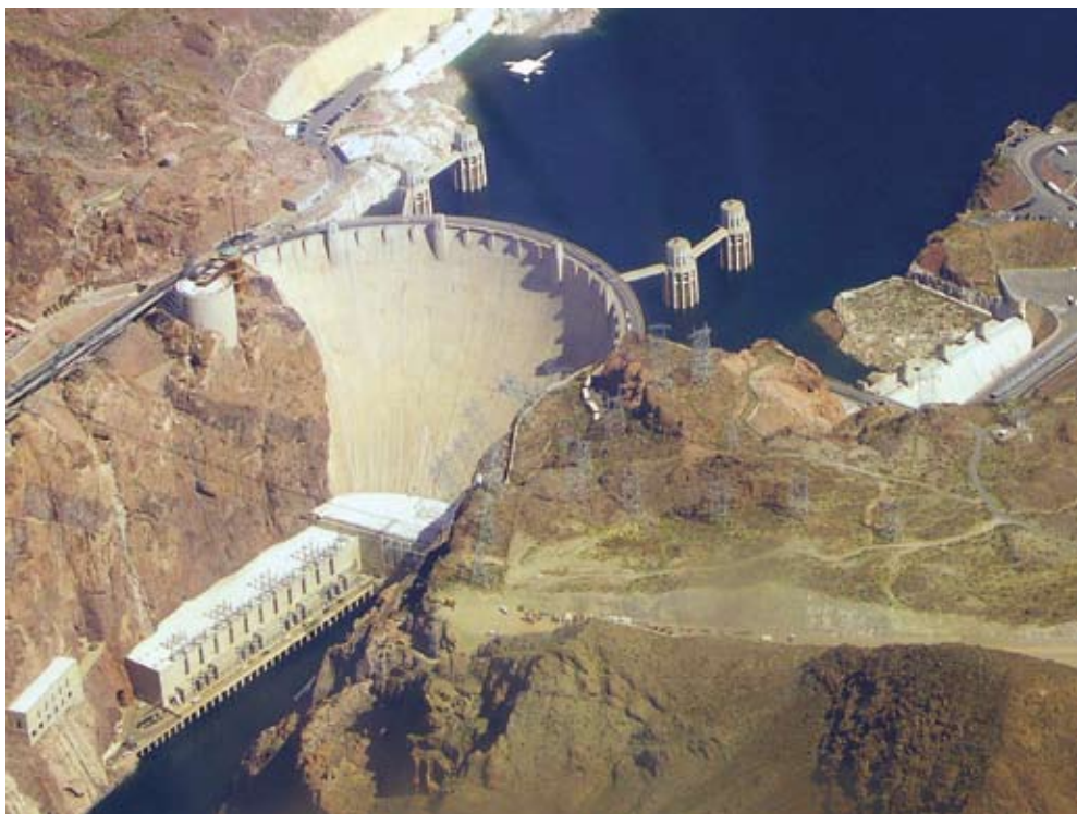
Along with the rest of the world, Endersbee was inspired by the Roosevelt-era great projects. Here, Hoover Dam, built by the Bureau of Reclamation, is a National Historic Landmark and has been rated by the American Society of Civil Engineers as one of America's Seven Modern Civil Engineering Wonders.
