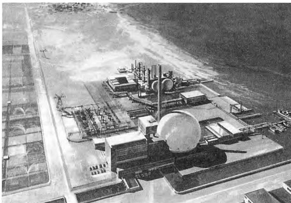
Nuclear energy will be used for many applications, such as desalination of seawater. This 1960's sketch is of a nuplex, an agro-industrial complex centered on a nuclear power plant. It is located on the seacoast, making possible the large-scale irrigation of farmland.
