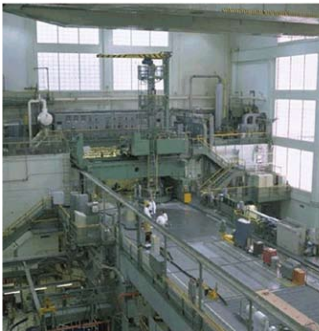
Inside the NRU Reactor at Chalk River, Canada, where MDS Nordion irradiates HEU targets to produce medical isotopes.
