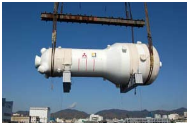
A nuclear steam generator in transport. Mitsubishi delivered two replacement steam generators for the San Onofre nuclear plant in California in February, each weighing 580 metric tons and housing about 10,000 heat transfer tubes.
