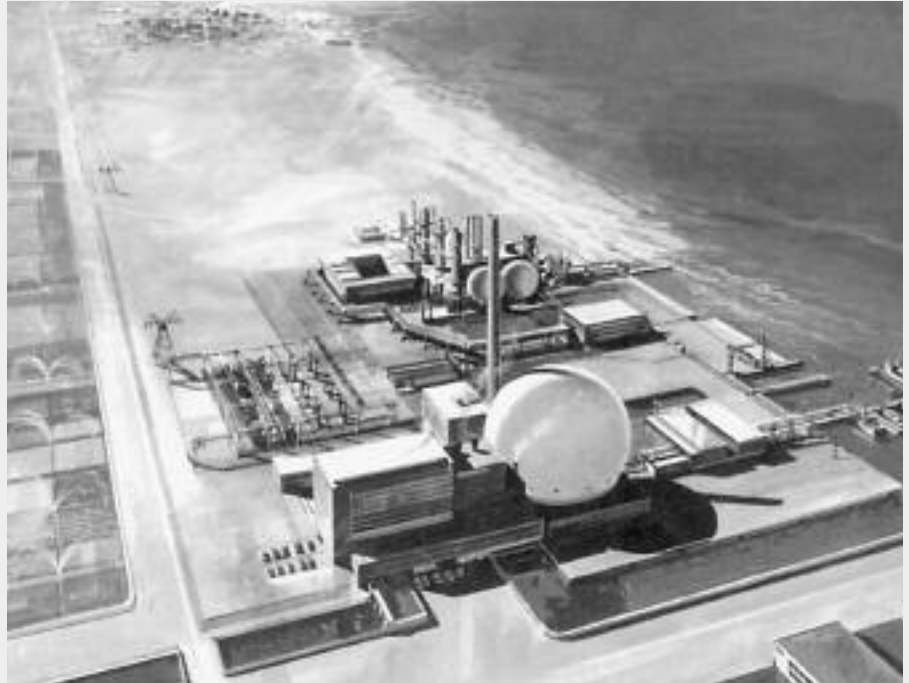
Artist's depiction of a nuplex, a nuclear-centered agro-industrial complex. This 1960s design was located on the seacoast for the purpose of desalinating seawater, as part of what Seaborg called a "food factory." In the "Atoms for Peace" optimism of the 1960s, it was assumed that nuplexes would be used throughout the world for development.
