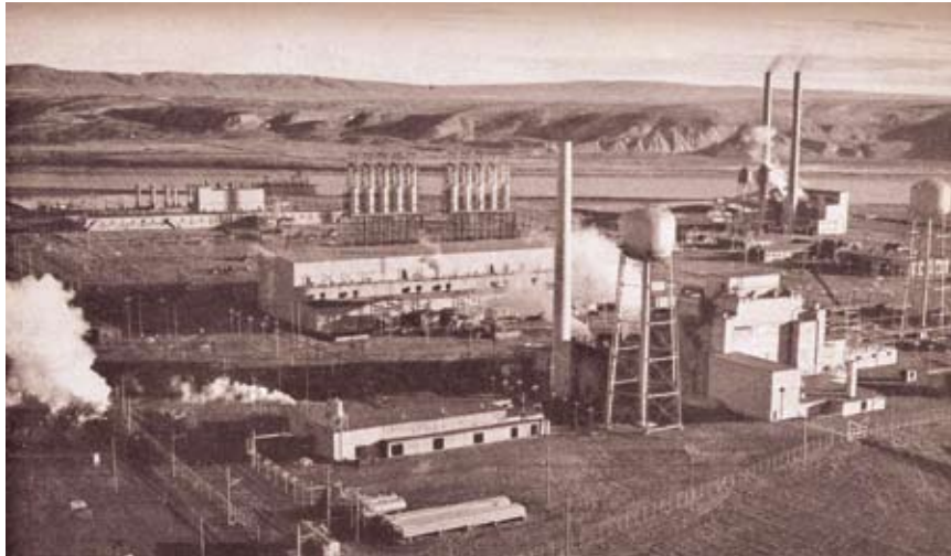
The F Reactor plutonium production complex at Hanford. The boxy building between the two water towers on the right is the plutonium production reactor; the long building in the center of the photograph is the water treatment plant
