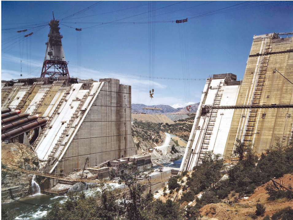
Shasta Dam under construction, June 1942.
