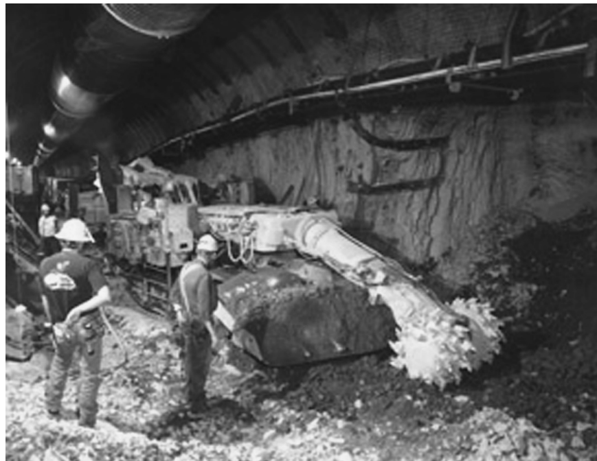
Excavation of one of seven alcoves in the main tunnel of Yucca Mountain, to investigate the mountain's geologic features. The nuclear renaissance in the United States does not have to wait for Yucca Mountain to be operational.
