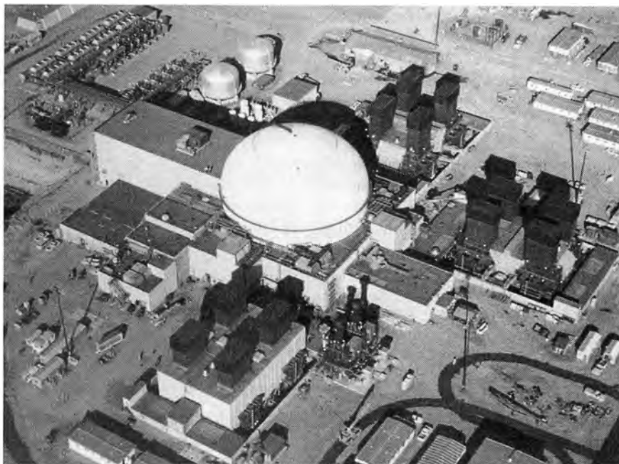
The Fast Flux Test Facility, at Hanford near Richland, Washington. The white dome is the containment building for the 400-megawatt test reactor.
