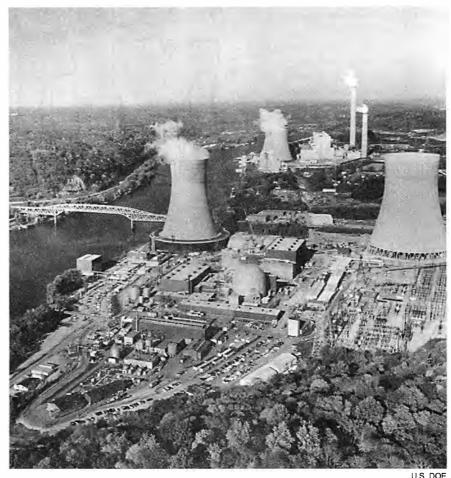
Shippingport Station, the first commercial nuclear power plant, located in Pennsylvania. During its operation, the reactor was fueled with three different types of cores, the last one being a light water breeder core.
