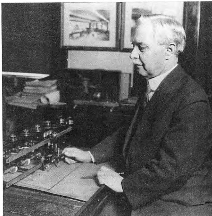
Dayton Miller at the Case School, with the Henrici harmonic analyzer, which he used earlier for sound and later for interpretation of interferometer data.
